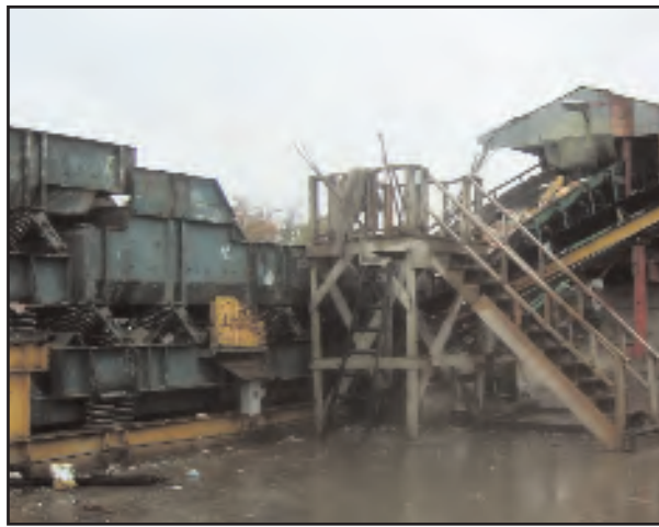
Once the large metal is removed, the remainder is dumped into the Action Screener and then conveyed up to the picking line.
